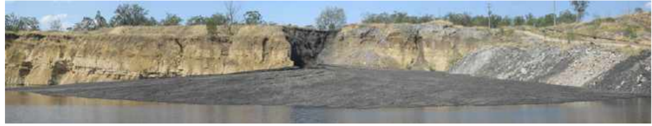
Figure 11. Pumped co-disposal of combined coal tailings and coarse coal rejects
